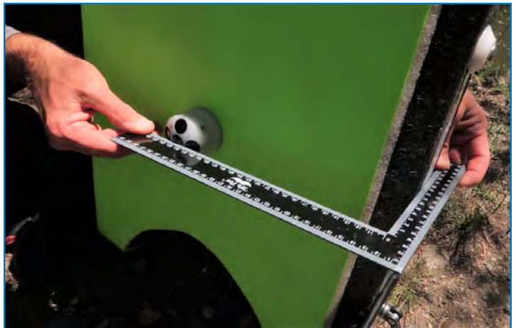
Figure 7. Lining up a carpenter square to the vertical beam.
